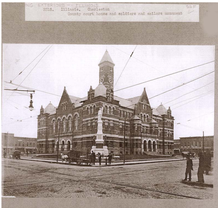
The current Coles County Courthouse, 1898-present
